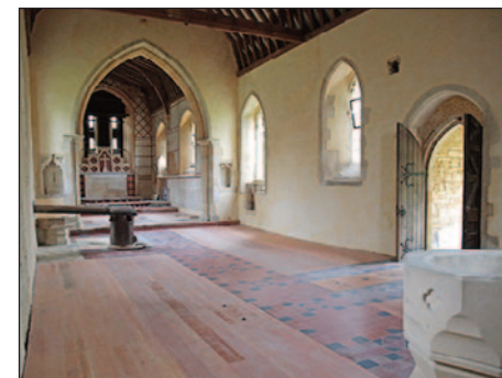
▼ The FoFC took ownership of St Denis’ in 2016, putting in a new floor and windows and, in 2022, replastering much of the nave.
