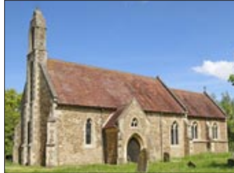
▲ St Denis' church, East Hatley in 2022: a handsome building made largely of fieldstones and now owned by the Friends of Friendless Churches, which is safeguarding it in perpetuity.
