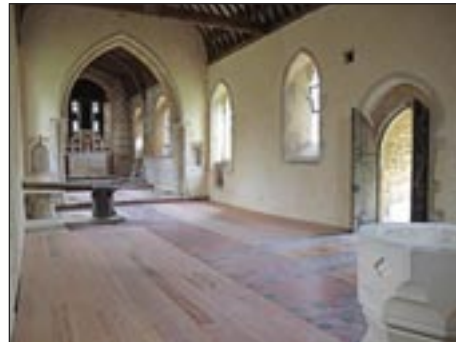
▼ The FoFC took ownership of St Denis' in 2016, putting in a new floor and windows and, in 2022, replastering much of the nave.
